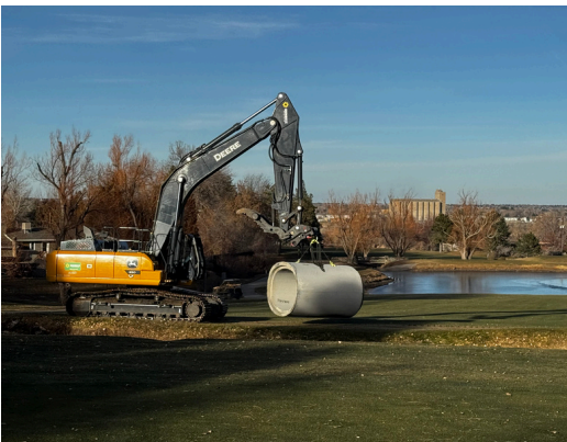
Rolling Hills Culvert Transport
