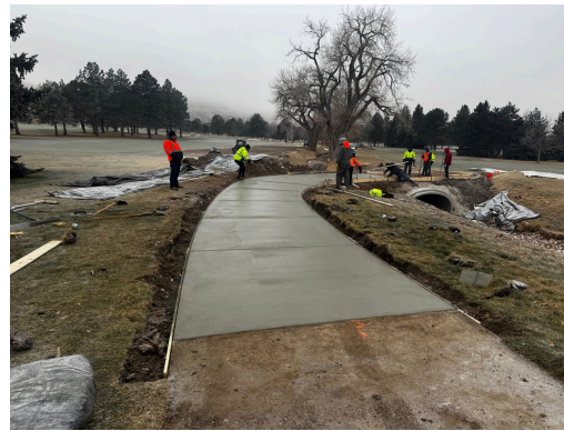
Rolling Hills Culvert and Concrete Repair
