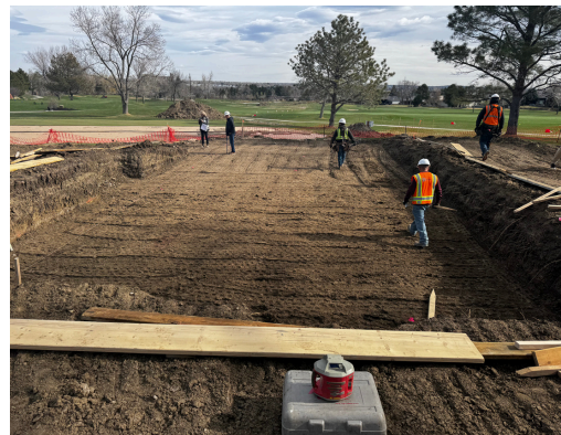
Rolling Hills New Comfort Station Build
