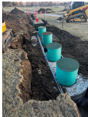
Rolling Hills Wastewater Treatment Install
