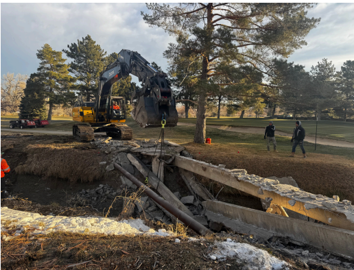
Rolling Hills Bridge Removal
